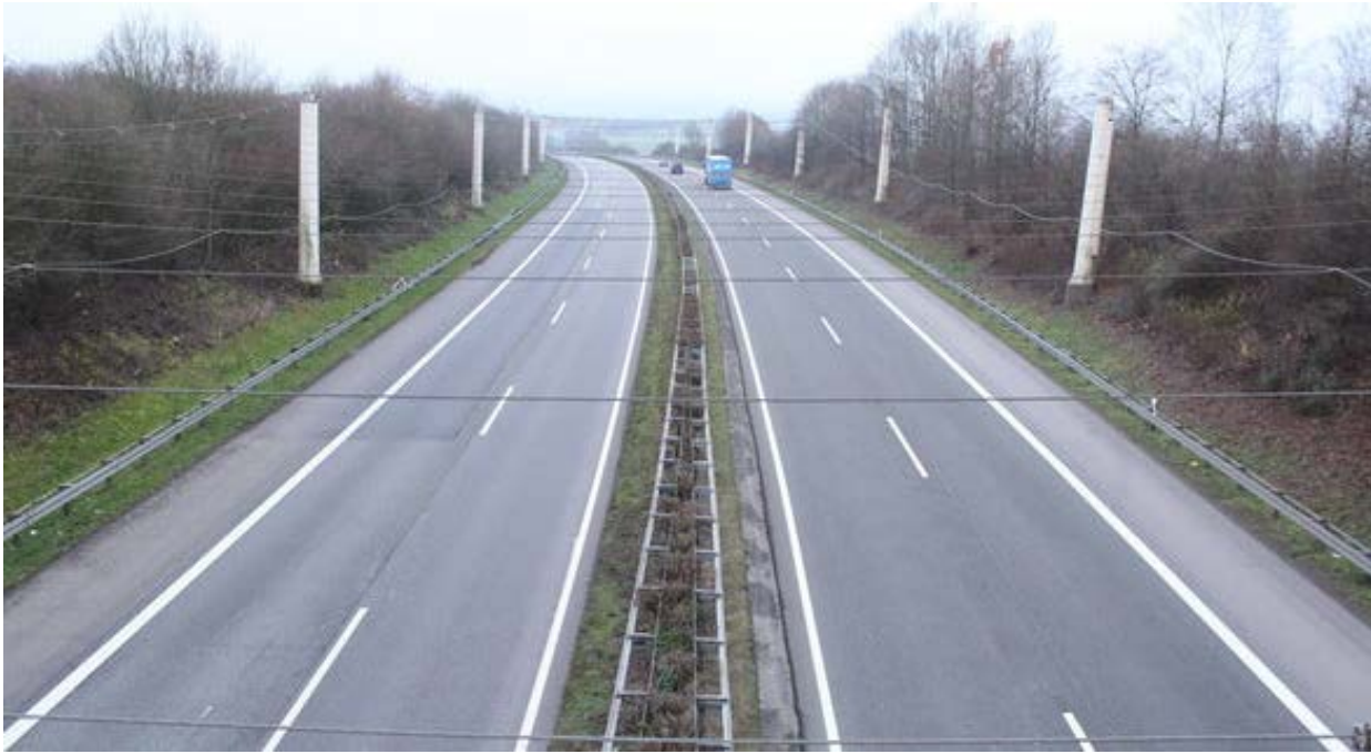
The Heusweiler Motorway Faraday Cage
